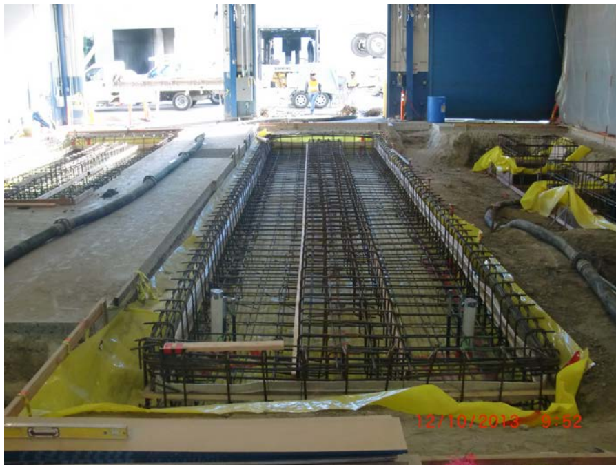
4. Reinforcing Steel Placement in Building A Bus Lift Pits.
